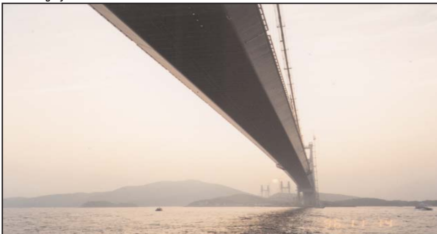
Figure 2: Lantau Fixed Crossing - Weather and Structural Health Monitoring System
